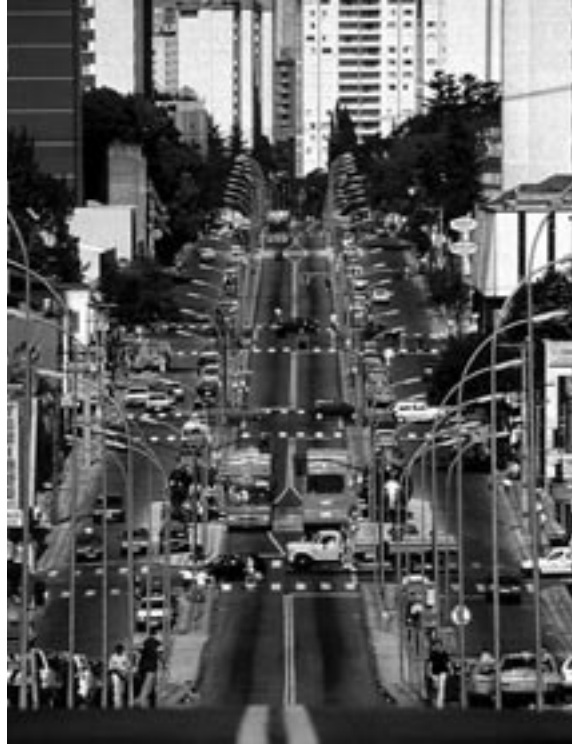
Curitiba, Brazil. View of main artery, showing central dedicated bus lanes that facilitate high-speed surface transit, a less-expensive alternative to an underground subway system.
