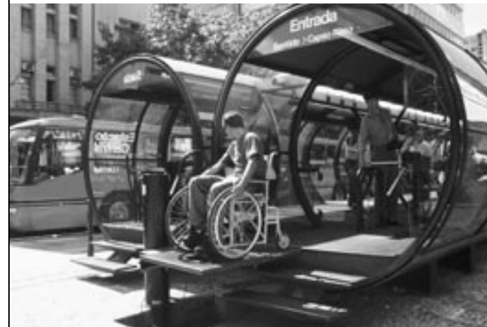
Left View of bus boarding tubes in Curitiba. Fares are paid on entering boarding tubes, which are elevated to bus entry level. Elevator platform raises wheelchair bound riders to door level before bus arrives. Both of these devices speed the transit time for riders.
