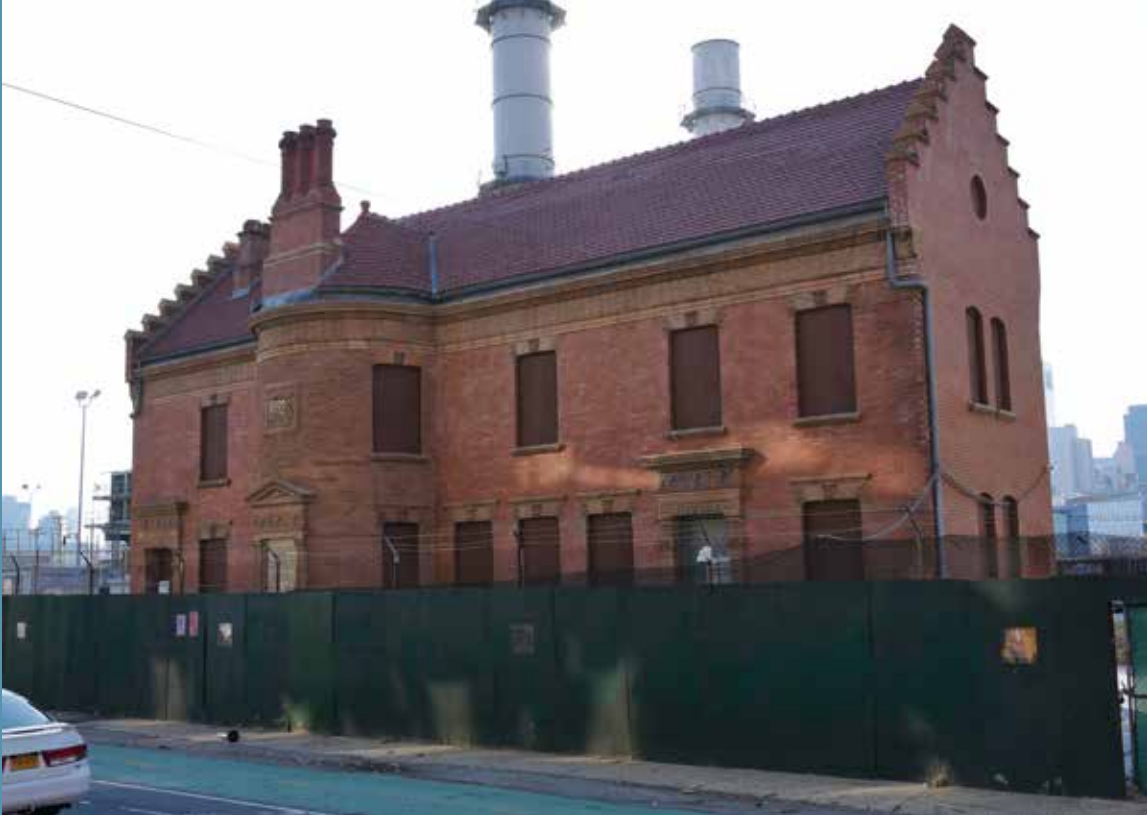
View of existing historic building adjacent to site
