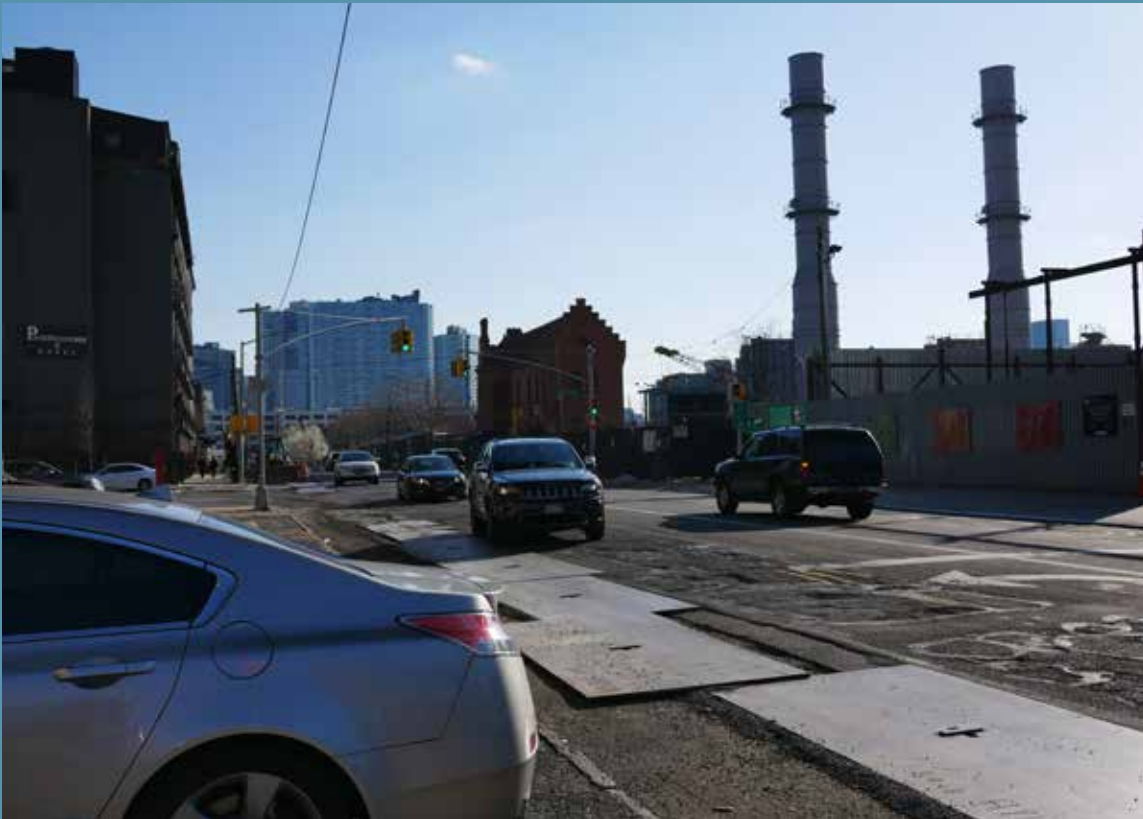
View of site from north
