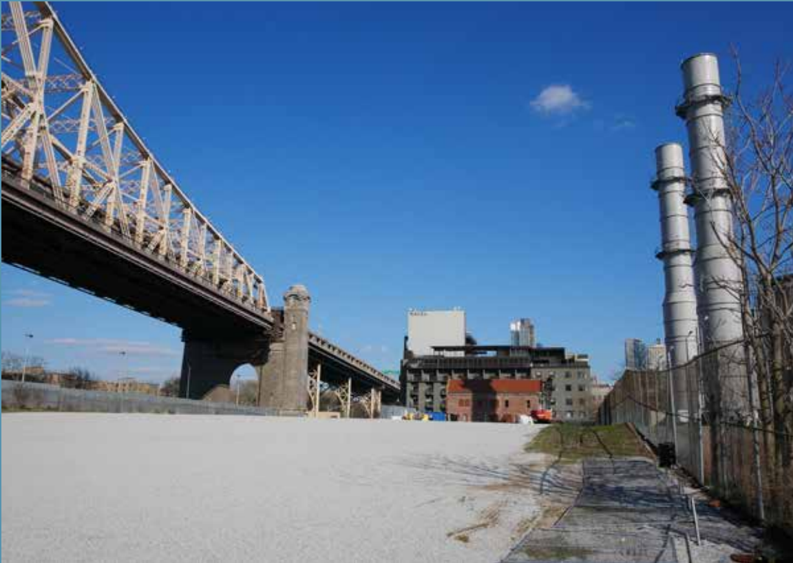
View of site from waterfront, looking east
