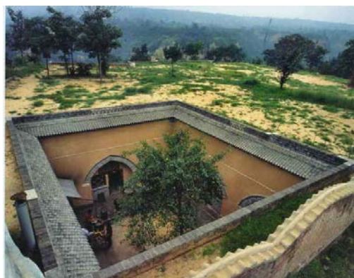
Figure 2 Sunken courtyard space of underground dwelling
